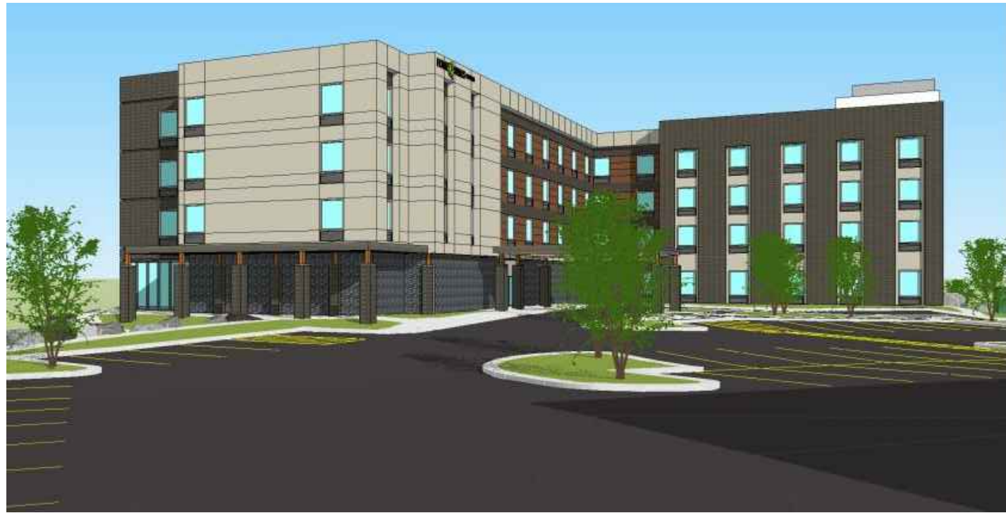
① WEST GROUND VIEW
